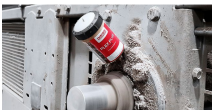
Lubrication of flange bearing on a conveyor
