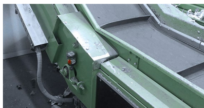
Bearing lubrication on a conveyor belt
