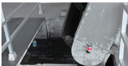
Lubrication of chain guide rollers
